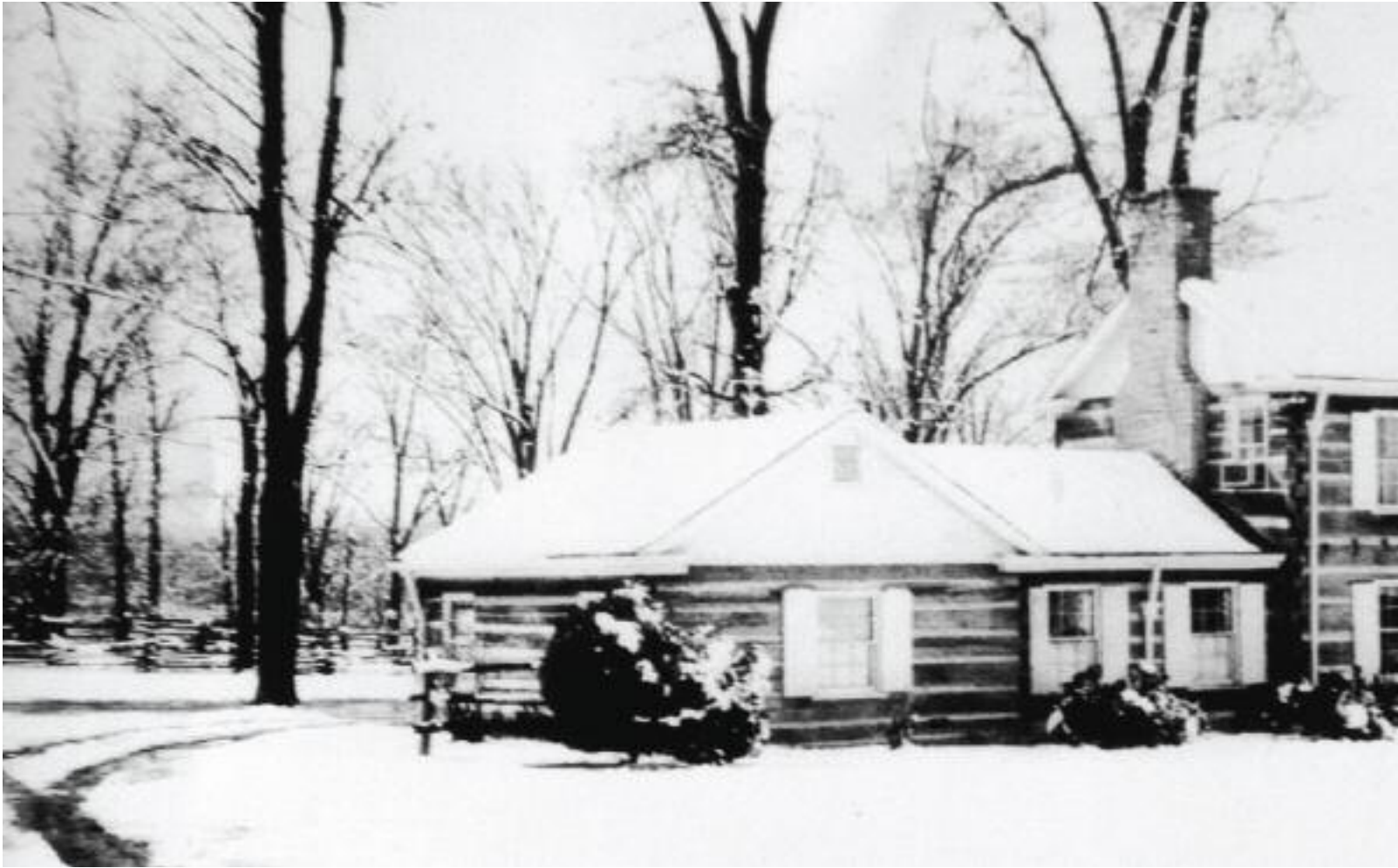
Hundred Oaks, the log house on Thompson Lane that was Carolyn Suschnick's girlhood home.
