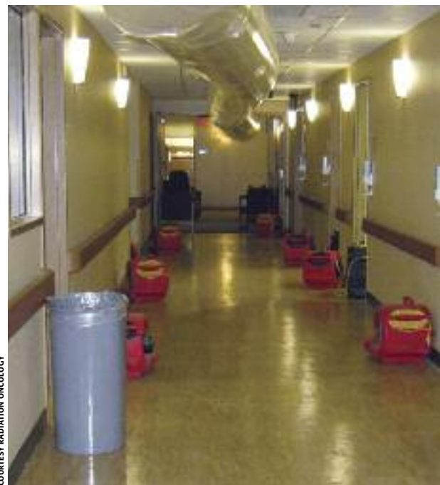
Fans were deployed all over the flooded basement areas to help quick drying.
